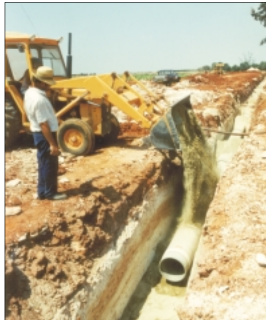
Laying of pipes at Kokkinokhoria
