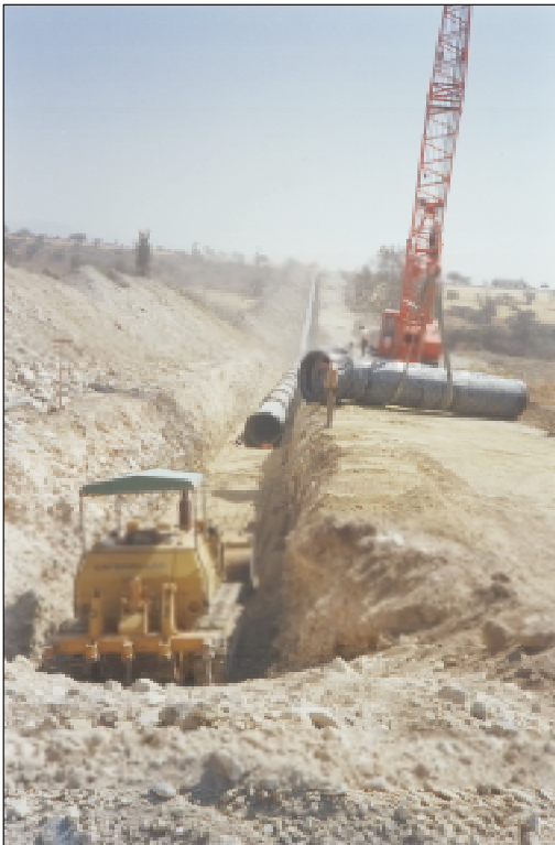
Laying of the main conveyor
