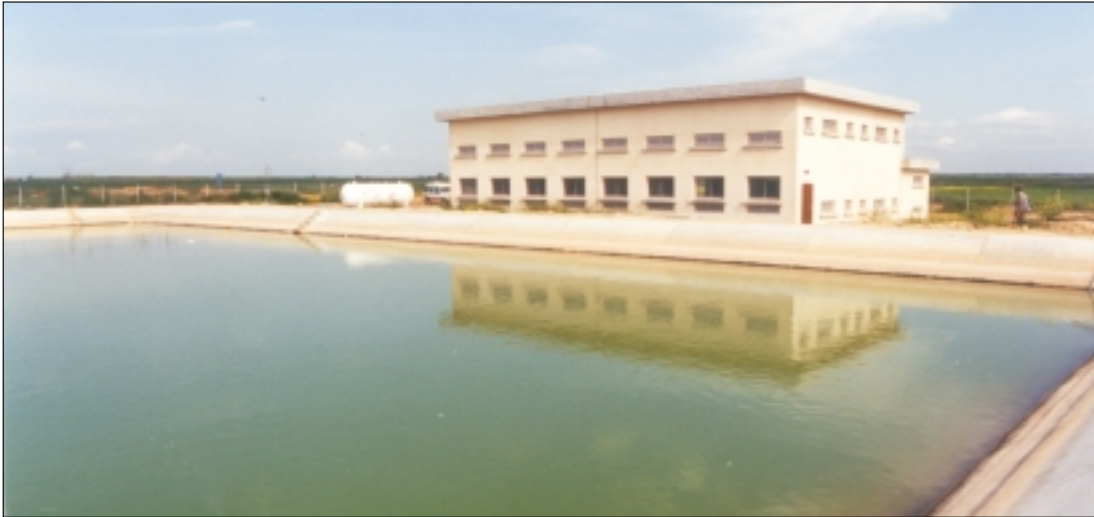
Central Distribution Point at Kokkinokhoria
