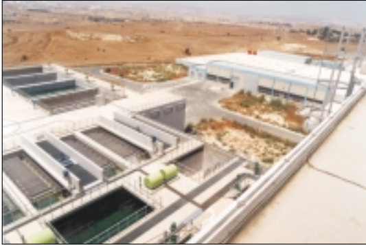
Tersephanou Water Treatment Plant
