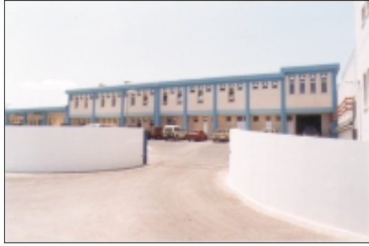
Administration building - Tersephanou Water Treatment Plant
